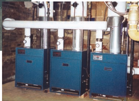
These 1,281 MBH hot water boilers (above) were installed and serviced by August Winter & Sons to meet the strict needs of a museum. Smaller boiler systems like this church retrofit (right) are routinely handled everyday by August Winter.
